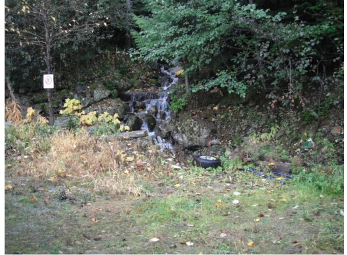
Photo 2. Tributary flowing southeast to northwest through the second culvert crossing at the driveway entrance. October 26, 2010.
